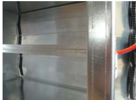
Detail FloXact® multipoint, averaging air flow sensor
