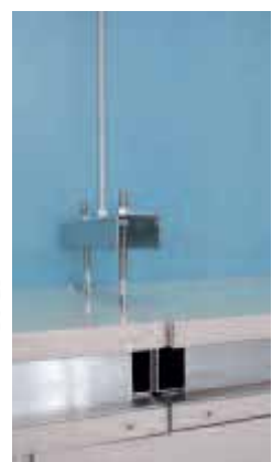
Wall/ceiling panels connection. Ceiling invisibly suspended.
